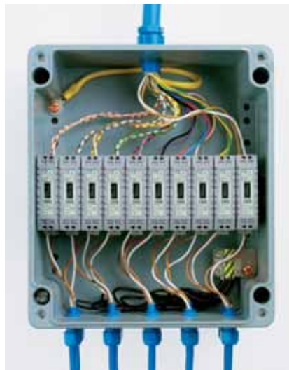
Figure 2. „Intelligent terminal“ in the field instead of a transmitter increases packing density.
